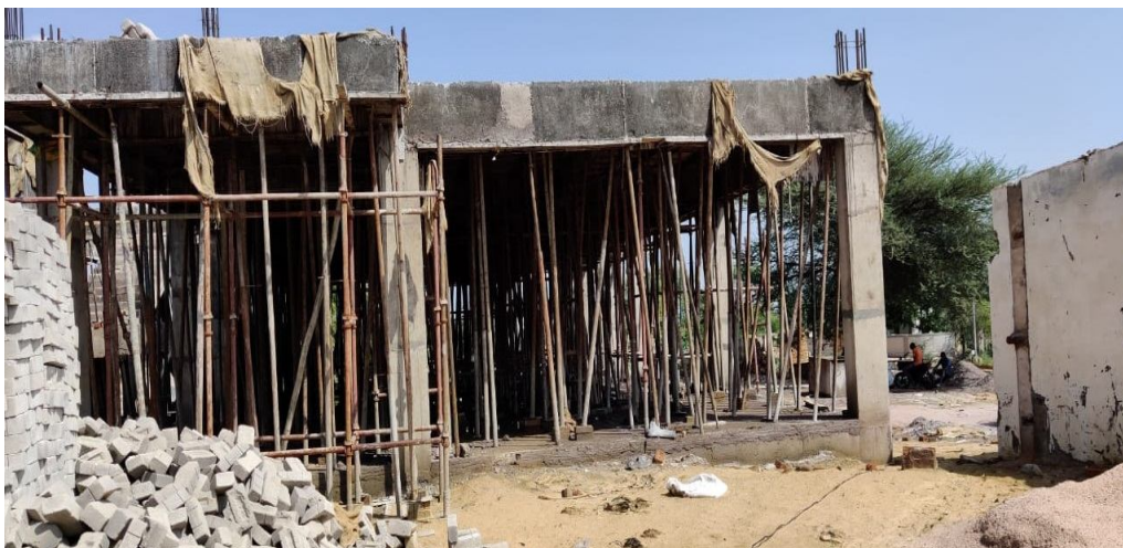
CANTEEN UNDER CONSTRUCTION
